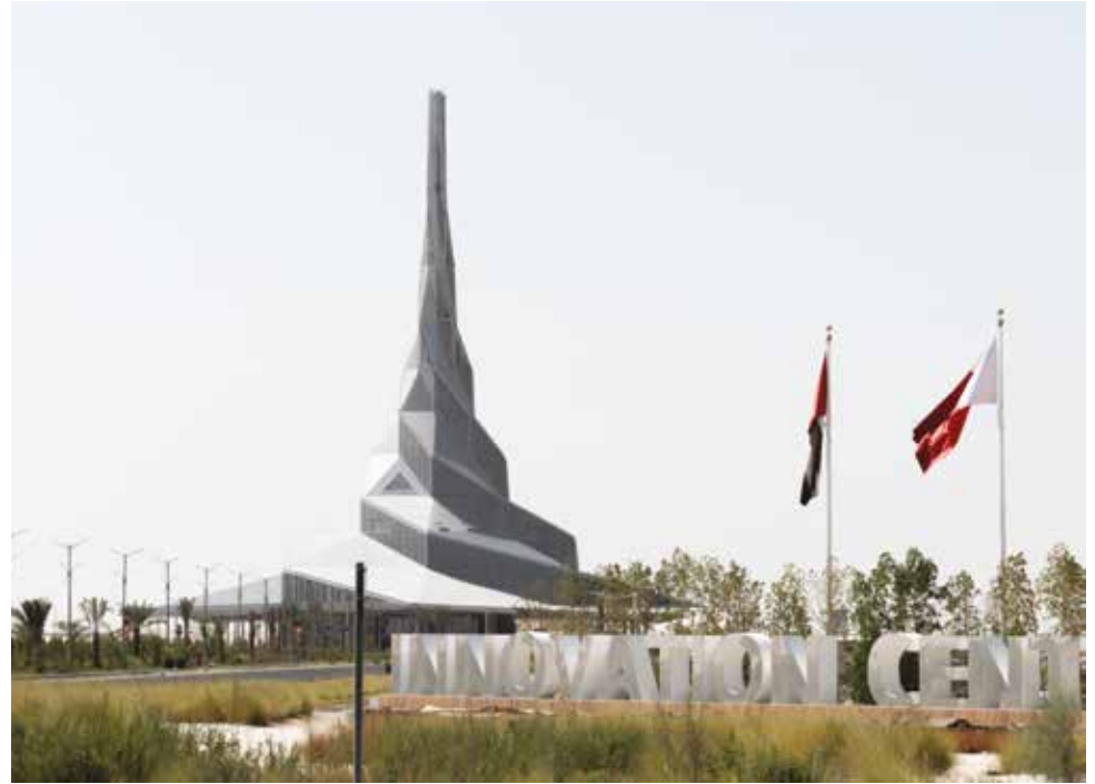
Solar Innovation Tower - AL Qudra-Dubai Client - Dewa
