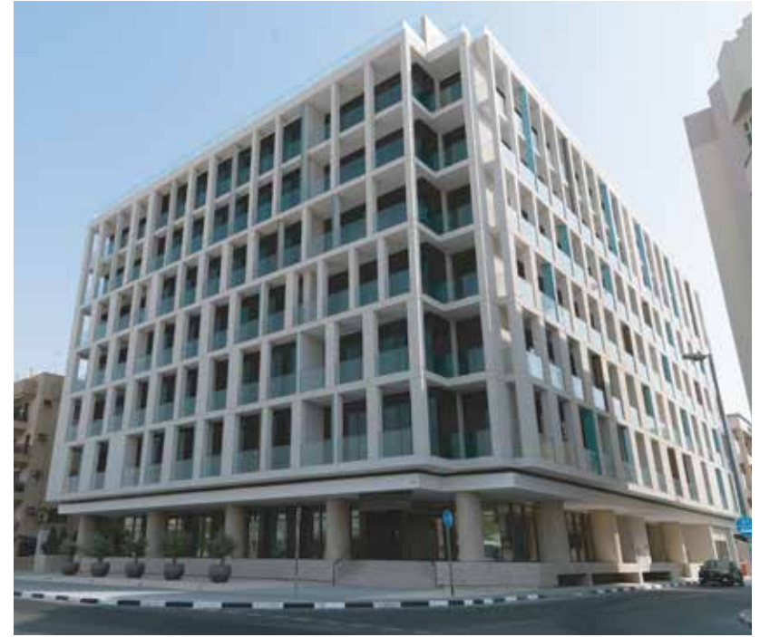
Lootah Building - Al Hamriya-Dubai Client - Lootah Family
